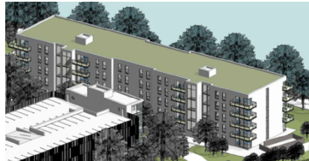
Figure 7.2 - Image of the Residential Building
